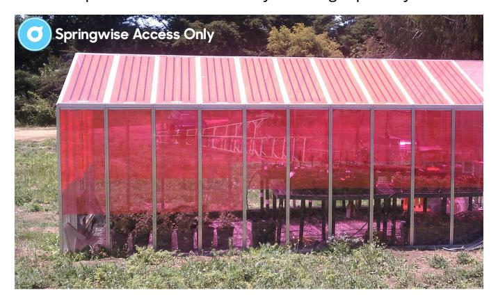
We have already seen <u>solar panels that work in the rain</u>, and now <u>Soliculture</u>'s LUMO solar electric panels are making greenhouses more profitable and energy efficient. LUMO panels convert green light to red, the color that plants use most for growth. By converting colors, rather than filtering them out, the panels have more light available for electricity production.
